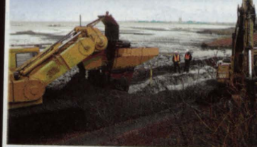
Impermeable trench using ORGANOCLAY® Organic Absorbent Media
